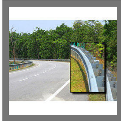
W Beam Crash Barrier
