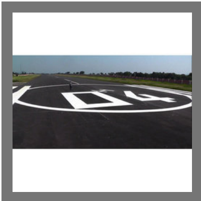
Thermoplastic Road Marking Work
